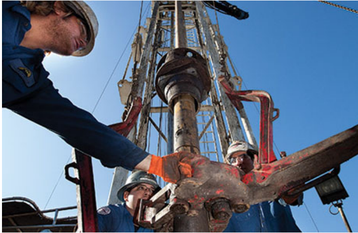
Signal Hill Petroleum crews working on an oil well near Walnut Avenue and 29th Street in Signal Hill. (Photograph by the Business Journal's Thomas McConville)
